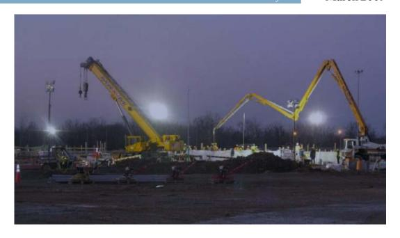
Getting a break in the weather, BGCAPP construction crews completed two concrete pours in February on the Munitions Demilitarization Building (MDB). Work on each of the pours began around 4 a.m. Between the two pours, over 600 cubic yards of non-blast concrete was placed in the MDB, the BGCAPP's main processing building.
